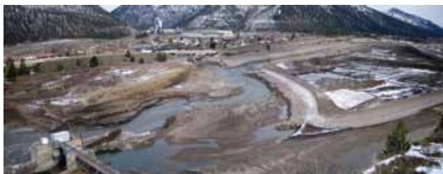
(Top) Shaded-relief image of Clark Fork arm of Milltown Reservoir, where colored areas show area and varying depths of post-dam breach scour from the reservoir. (Bottom) Milltown Dam and Reservoir, from similar perspective as photo at top left of page, one day after breaching of the dam in March 2008 but prior to complete removal of the structure.
